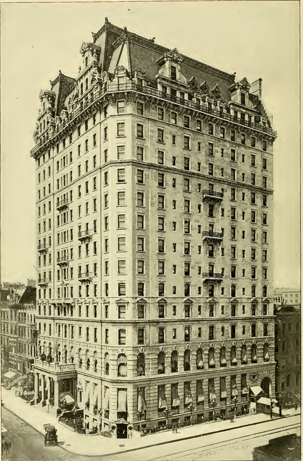
Manhattan Hotel, New York. 1300 H.P. Babcock & Wilcox Boilers.
